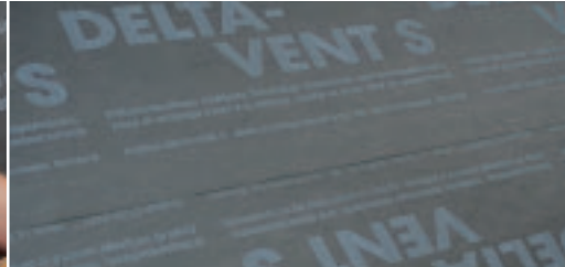
Product identification markings serve as guide for overlap edge.
