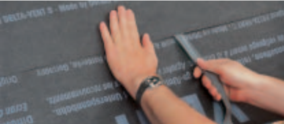
Wind-tight overlap seams with DELTA®-VENT S PLUS.
