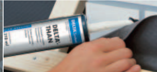
Secure connections with DELTA®-THAN sealant.
