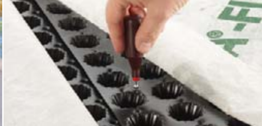
Joining sheets with DELTA®-FLORAXX connecting elements.
